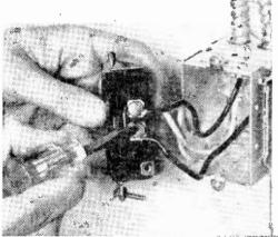
Soldered splices aren't used much any more. Circuit is completed by the connection between screw terminals.
