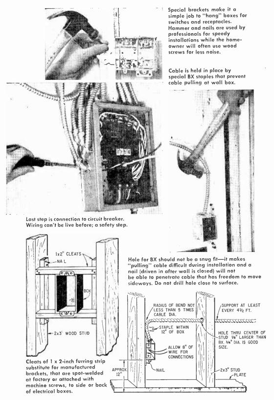
How you Add-A-Outlet depends on location of existing wiring and outlet boxes. The connections are simple. Running the cable through finished walls and ceilings can be a big problem.
