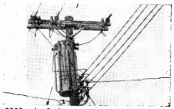
2300-volt, 3-phase power arrives on upper wires. Pole transformer drops it to 120/ 208 and feeds homes via lower four wires.
