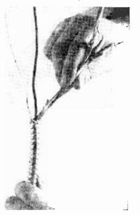
Remove kraft-paper wrap but not ground lead—bend back; wrap around cable; secure in clamp.
